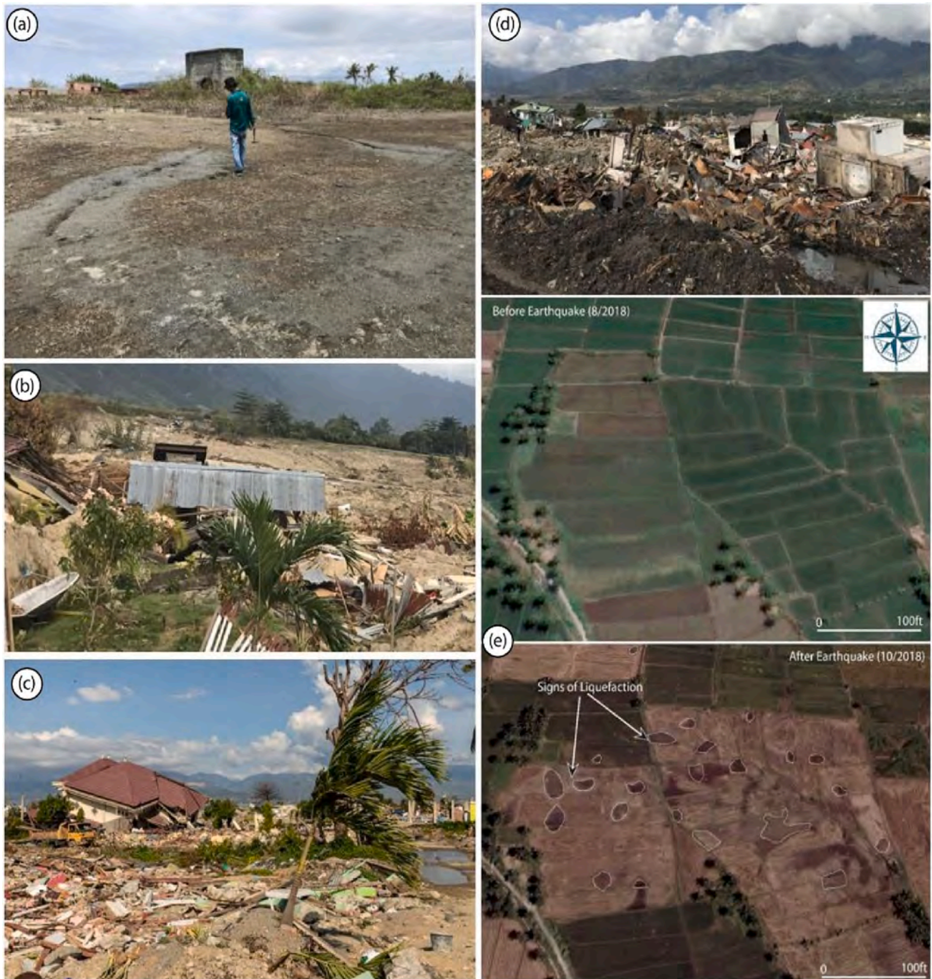
Fig. 13. Field and satellite photos showing evidences of liquefaction and damaged houses due to liquefaction induced lateral spreading around Petobo, Sigi Biromaru and Sibalaya (Google Earth image source: https://earthengine.google.com/ ).
