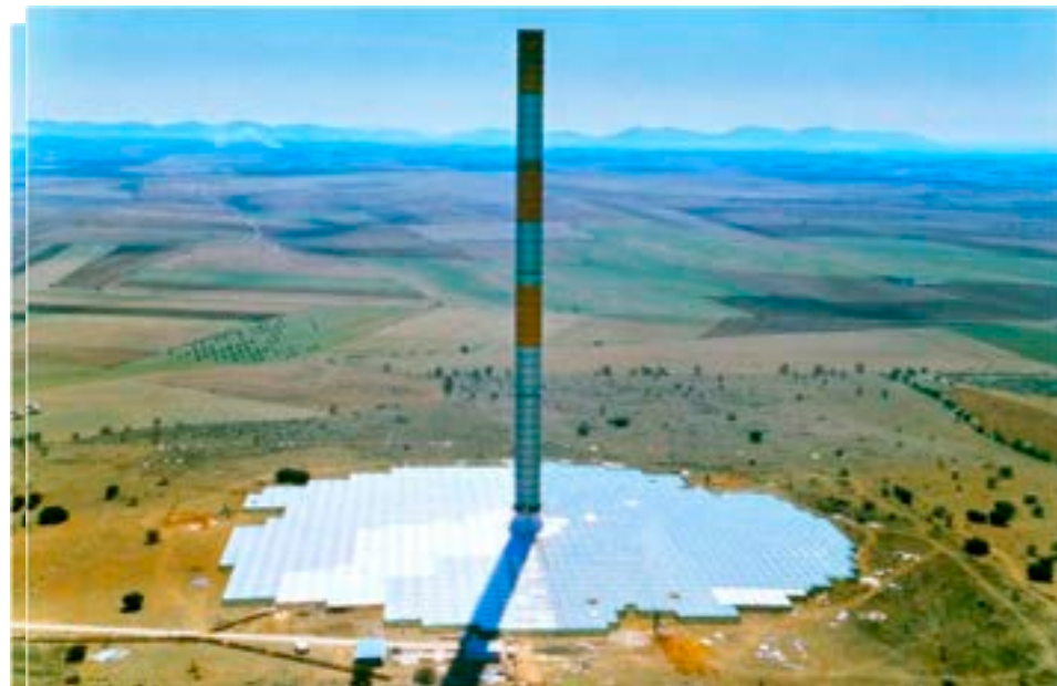
Figure 2. Manzanares Solar Chimney Test Facility, established in 1982 in Spain [8]. (Adapted with permission from ref. [8]. Copyright 2019 Elsevier.)
