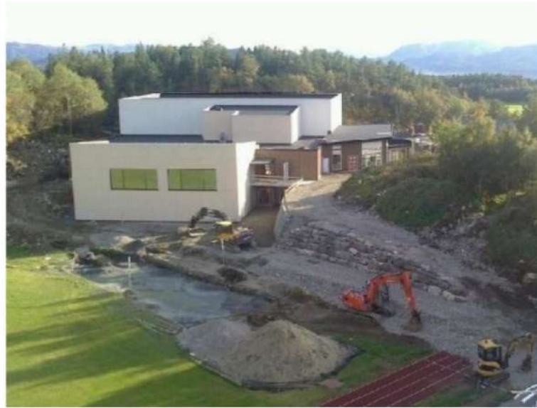
Figure 3. The northern façade of the building.
