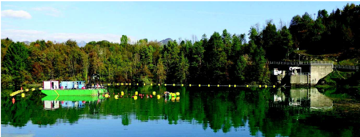
Figure 5.3. Hydraulic dredging. The sediment mixed with water was discharged through the surface spillway to the Ambiesta River.
