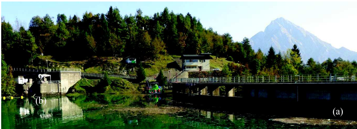
Figure 5.2. (a) Ambiesta dam and (b) its surface spillway (outside the body of the dam).
