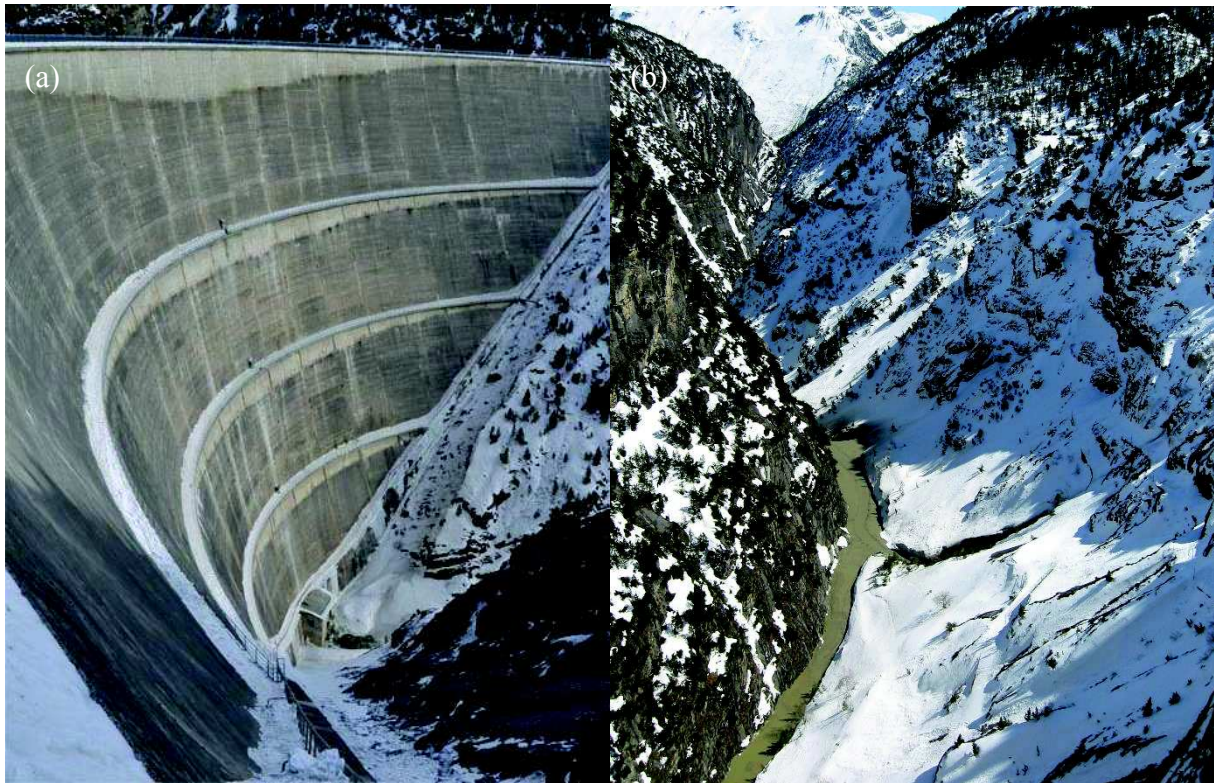
Figure 3.5. (a) The bottom outlet of Cancano Reservoir and (b) the River Adda just downstream of the dam during the 2012 flushing operation.
