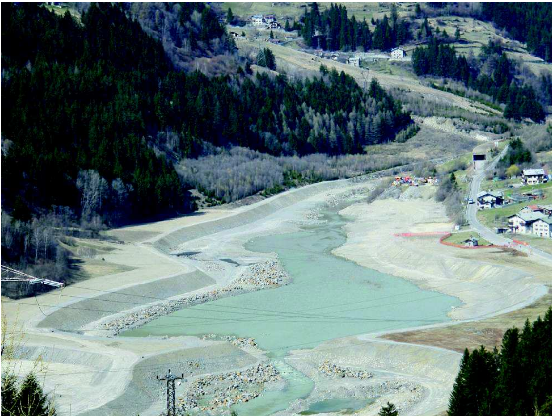
Figure 3.2. The instream settling basin (the Val Pola Pond) looking upstream before the 2011 flushing event.
