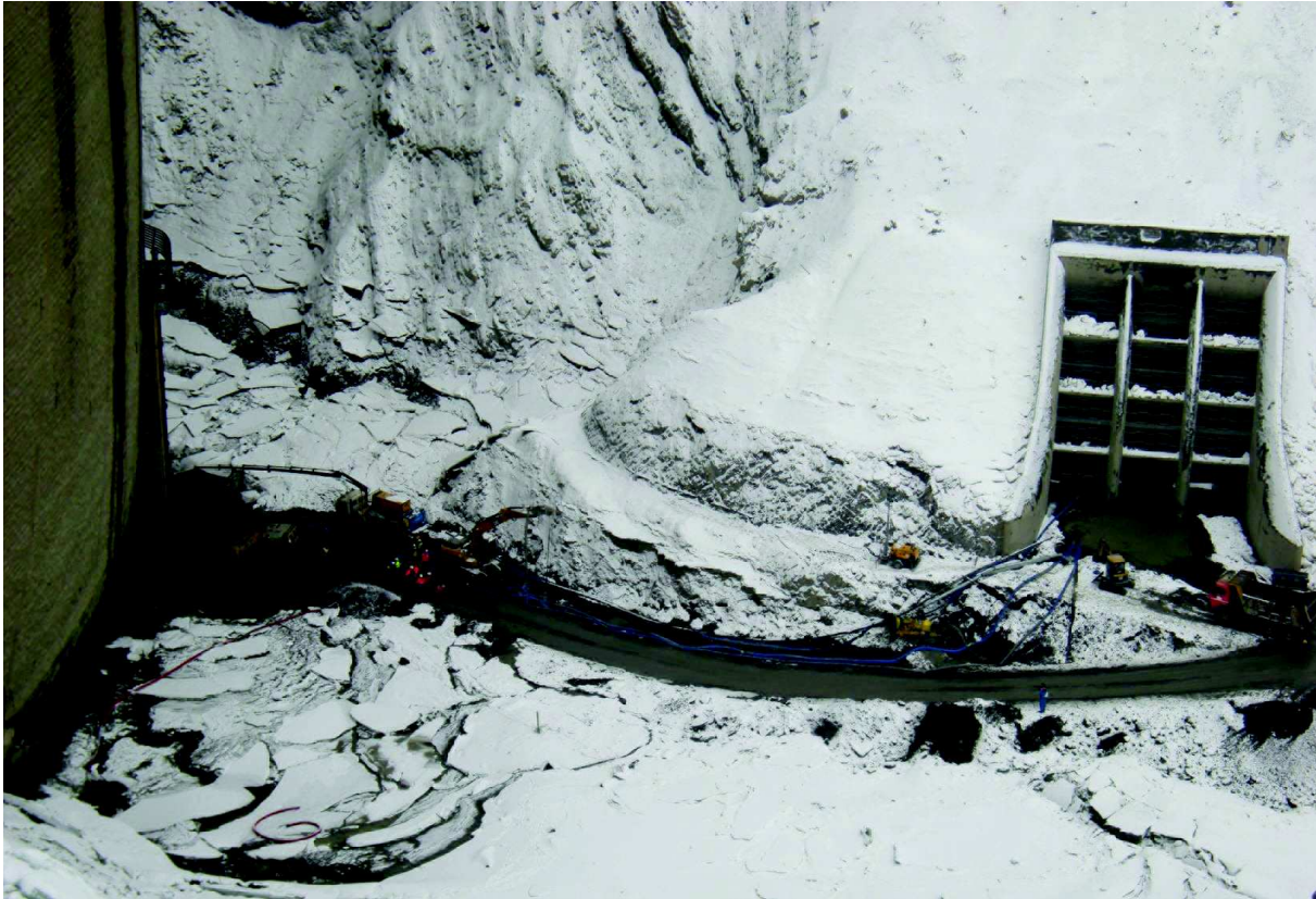
Figure 3.4. The Cancano Reservoir during the 2010 flushing event: earth-moving equipment working close to the upstream face of the dam can be seen on the left side of the photograph, the power intake on the right side.
