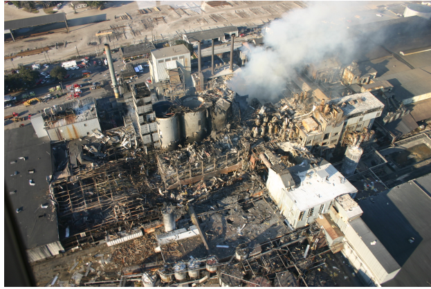
Figure 2.8: Picture of the Imperial Sugar plant after the accident (Source: CSB, official website)
