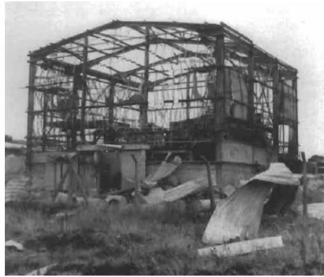
(a) Picture of the screen room after the explosion
