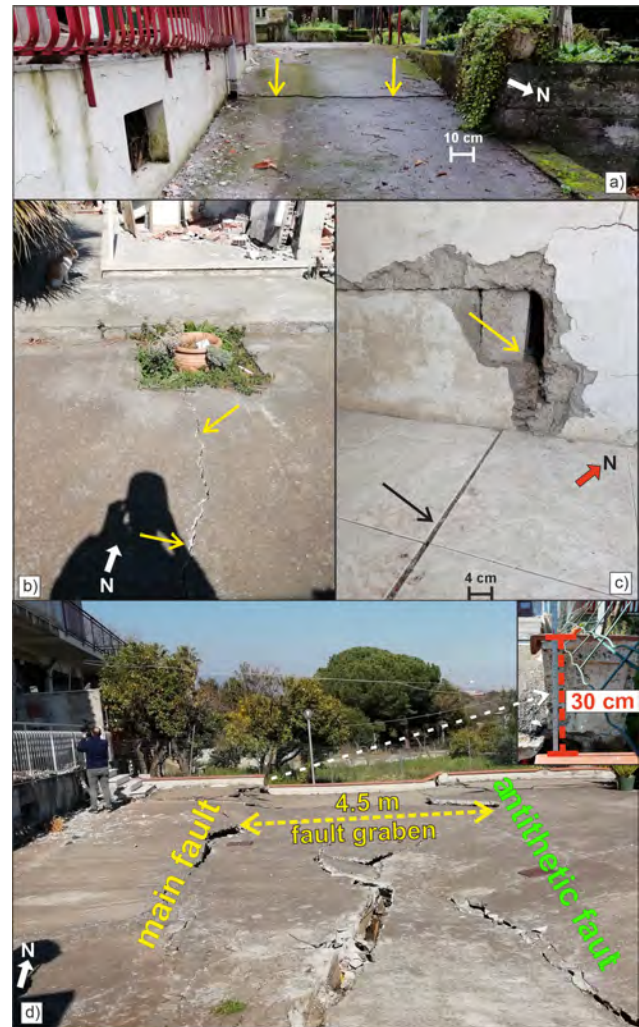
Figure 5. 26 December 2018 coseismic ruptures at Fiandaca trench site (see photos location in Fig. 4): (a) ground rupture along a private road with few cm of offset; (b) ground rupture which follows a damaged building wall, offset \sim 1 cm; (c) 1.5 cm horizontal offset between two floor tiles continuing into the wall; (d) fault graben on a private asphalt parking which extends over the wall and farmland. Photos taken on: 26 December 2018 (a); 22 January 2019 (b and c); 18 February 2019 (d).
