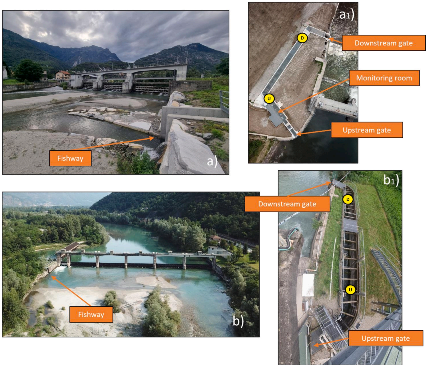
Fig. 2. Photos of the Tana (a) and Prata (b) dams with fishways, showing antennas placements (i.e., yellow dots: U = upstream antenna; D = downstream antenna), and details of the fishways (respectively a 1 and b 1 ).
