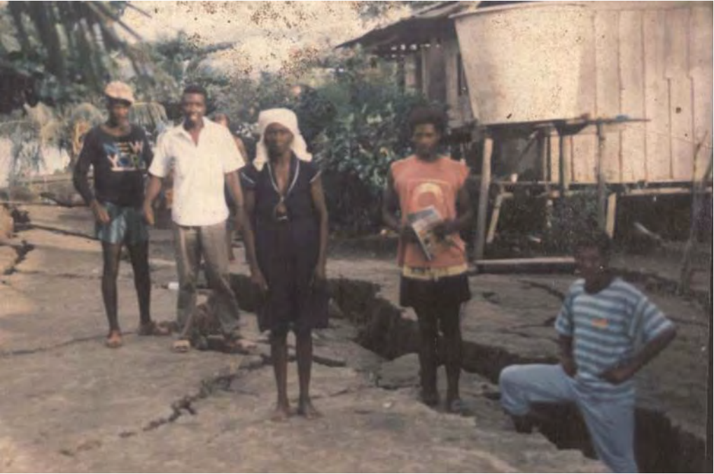
Fig. 7. Ground cracks induced by the Murindo events of October 1992 in Bojaya, (photo: S. Mosquera-Machado). For municipality locations, see Figure 3.
