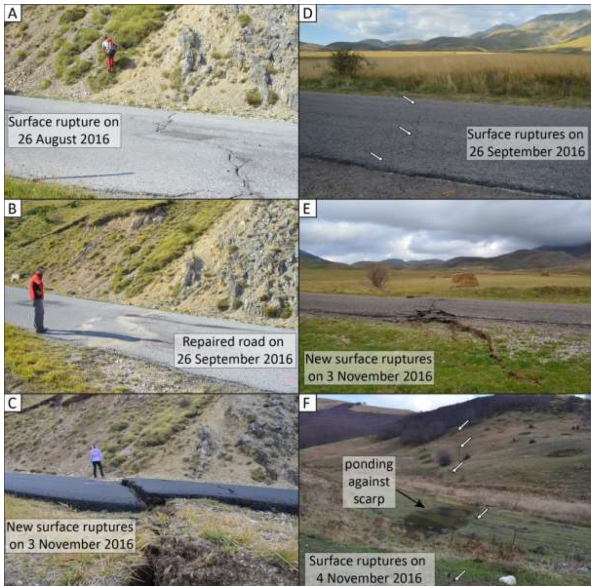
Figure 1: Earthquake environmental effects due to the 2016 earthquake sequence in Central Italy. A) Surface ruptures offset a road in the 24 August, 2016, Amatrice Earthquake ( M_w6.2 ). B) On 26 September, 2016, the road was repaired. C) On 26 October, 2016, the M_w6.6 Norcia Earthquake ruptured the same fault again and offset the re-paved road. T D) Surface ruptures in a road due to the Amatrice Earthquake. E) New surface ruptures were found to offset the road after the Norcia earthquake. This modern example illustrates the pitfalls related to interpreting geological data from palaeo-earthquakes. Looking back a couple of hundreds or even thousands of years, it will be hard or even impossible to distinguish the geological traces of individual moderate earthquakes within a seismogenic zone. Thus, primary offsets used for the reconstruction of palaeo-magnitudes may be misinterpreted. F) Uphill-facing vertical offsets due to the Norcia Earthquake led to ponding in the Castelluccio Plain (photo from 4 November, 2016). In the geological record of palaeo-earthquakes, such features might be preserved as anomalous fine-grained layers in the stratigraphy.
