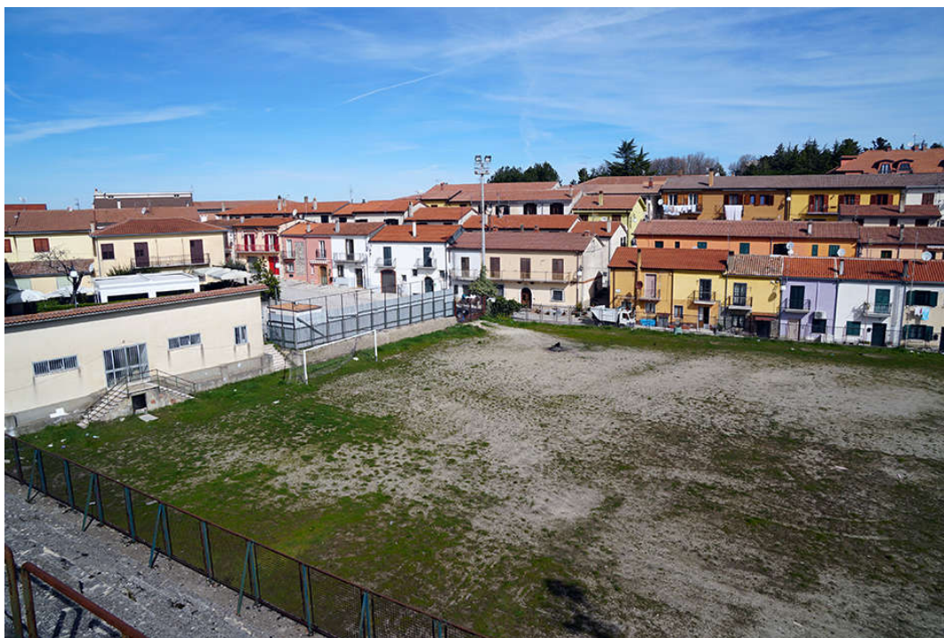
Figure 39. Sant'Angelo dei Lombardi: overview of new buildings and the football field (photos by [35,36]).
