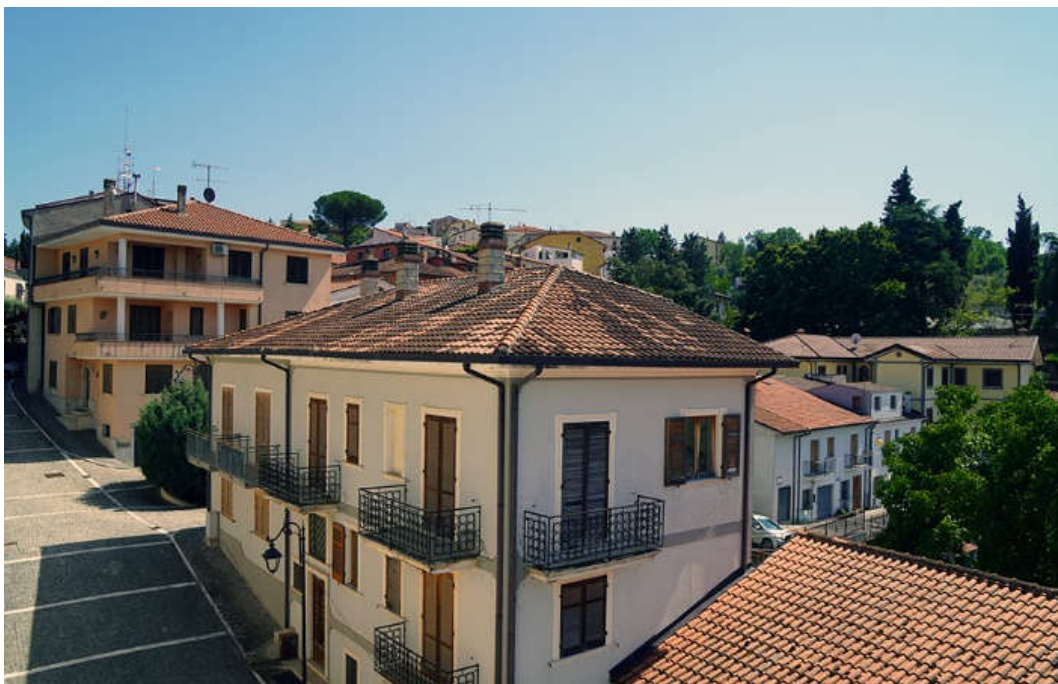
Figure 78. Torella dei Lombardi: details of the new buildings (photos by [35,36]).
