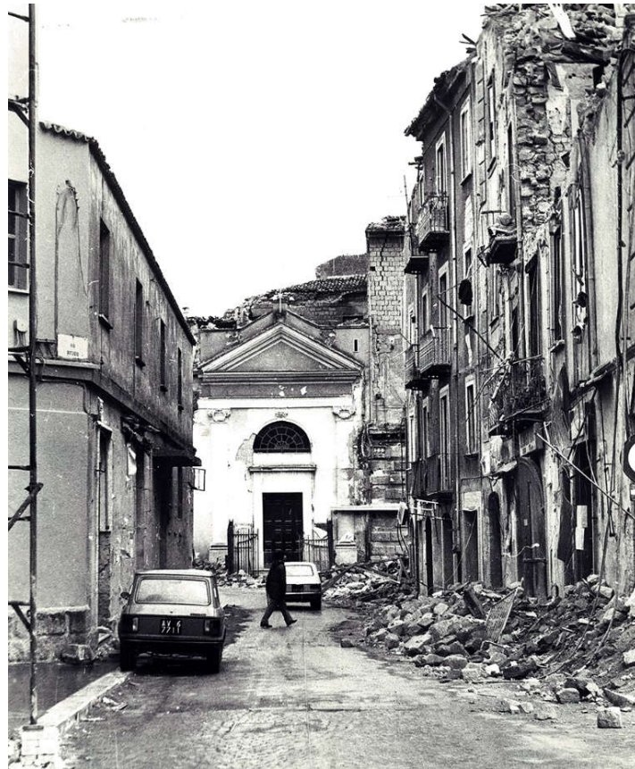
Figure 116. Avellino: Rifugio Street after 1980 earthquake (cortesy of F. Capossela).
