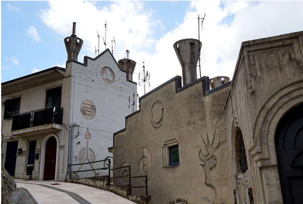
Figure 43. Balvano: the new buildings details of the architecture by R. Boffo and K. Eibl (photos by [35,36]).
