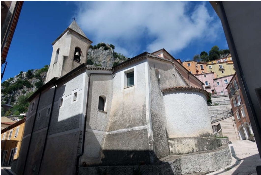
Figure 84. Colliano: detail of the restored historical centre (Church of Santa Maria del Borgo) (photos by [35,36]).
