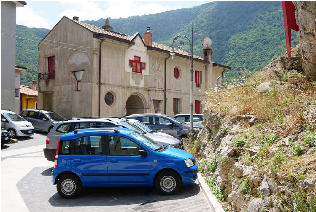
Figure 42. Balvano: the new buildings details of the architecture by R. Boffo and K. Eibl (photos by [35,36]).
