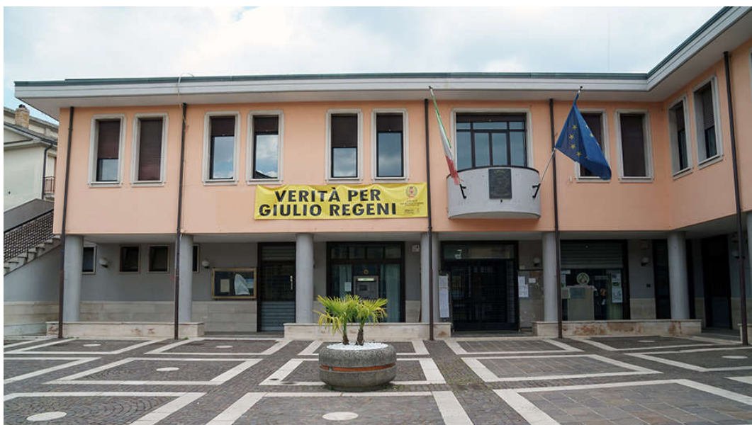
Figure 61. San Michele di Serino: the new municipal building (photos by [35,36]).
