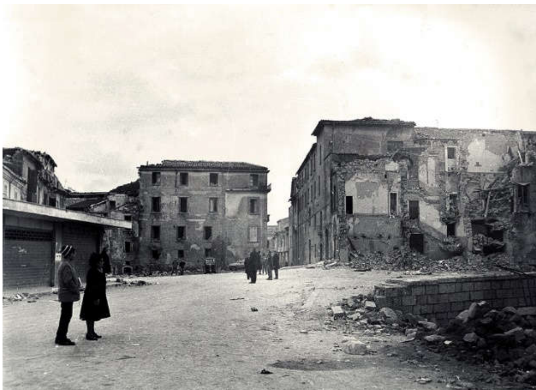
Figure 118. Avellino: “Piazza del popolo” after the 1980 earthquake (courtesy of F. Capossela).
