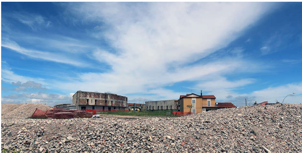
Figure 108. Bisaccia: the new village (Piano di Zona) with the remains of the new social housing still to be completed (Istituto Autonomo Case Popolari-IACP). A part of them has been demolished in 2020 (photos by [41]).
