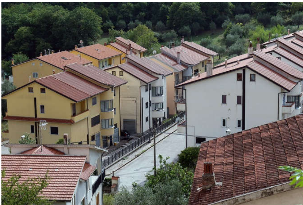
Figure 93. Salvitelle: details of new buildings (photos by [35,36]).
