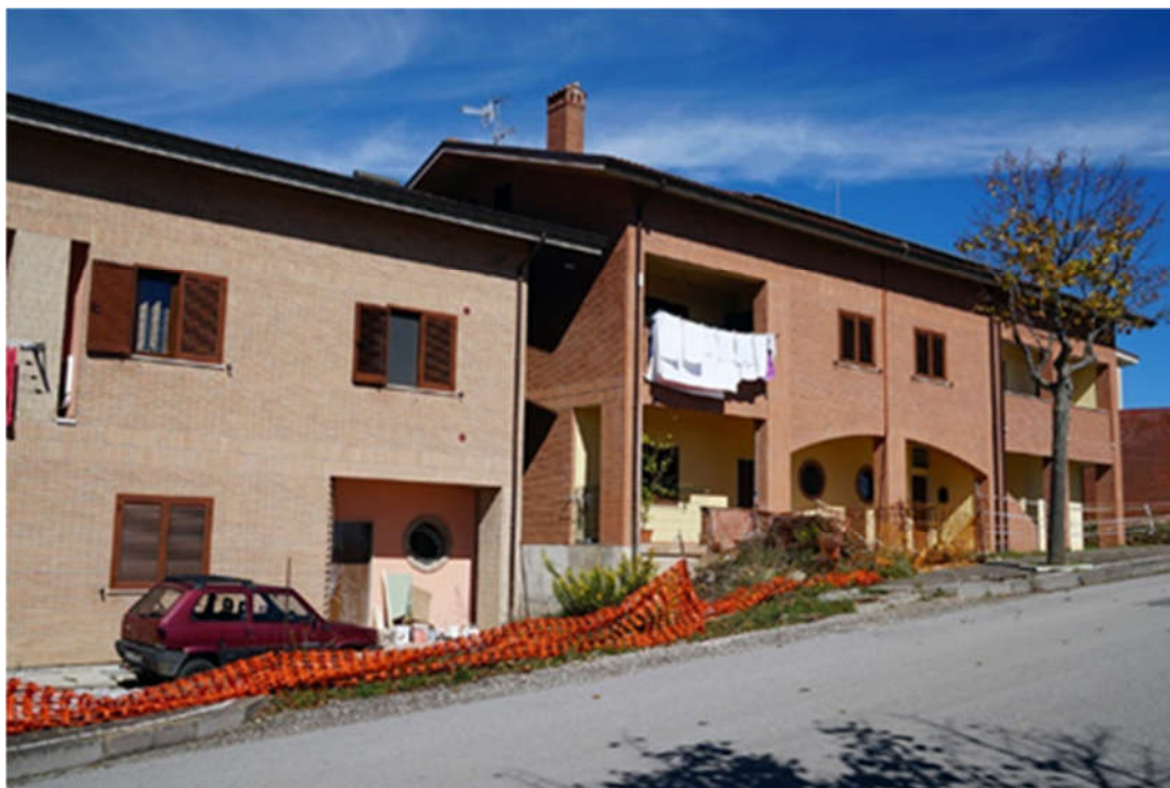
Figure 89. Romagnano al Monte: details of new buildings in the new town (photos by [35,36]).
