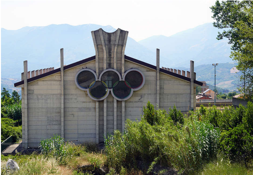
Figure 7. Castelnuovo di Conza: the new sports hall (photos by [35,36]).
