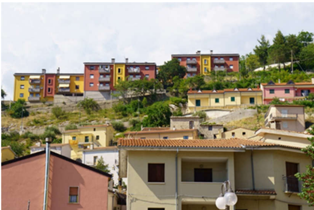
Figure 31. Santomena: a detail of the new buildings (photos by [35,36]).
