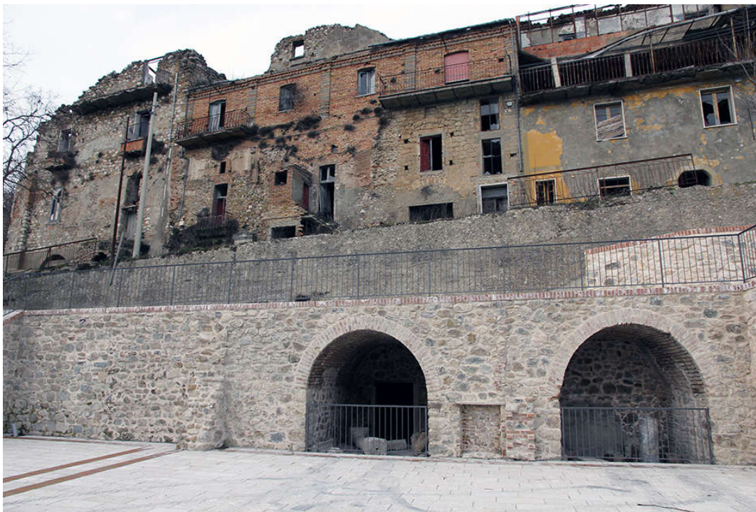
Figure 12. Conza della Campania: old village with ruins of houses after the 1980 earthquake (photos by [35,36]).
