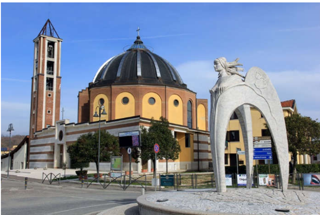
Figure 17. Conza della Campania: new village with the new Cathedral "Concattedrale di Santa Maria Assunta" in the center of village built after the 1980 earthquake (photos by [35,36]).
