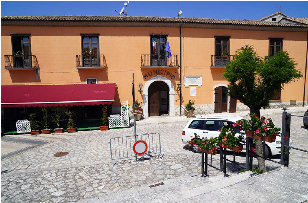
Figure 74. Guardia dei Lombardi: the new Town Hall of village (photos by [35,36]).
