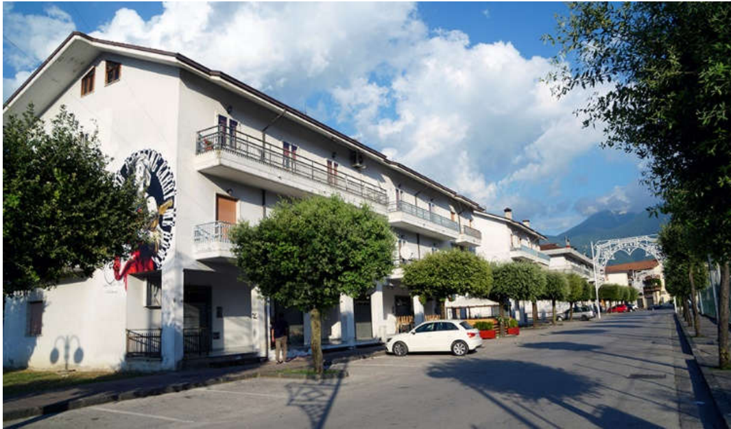
Figure 62. San Michele di Serino: new reinforced concrete buildings (photos by [35,36]).
