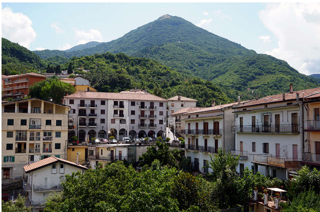
Figure 48. Calabritto: panoramic view of the village completely rebuilt (photos by [35,36]).
