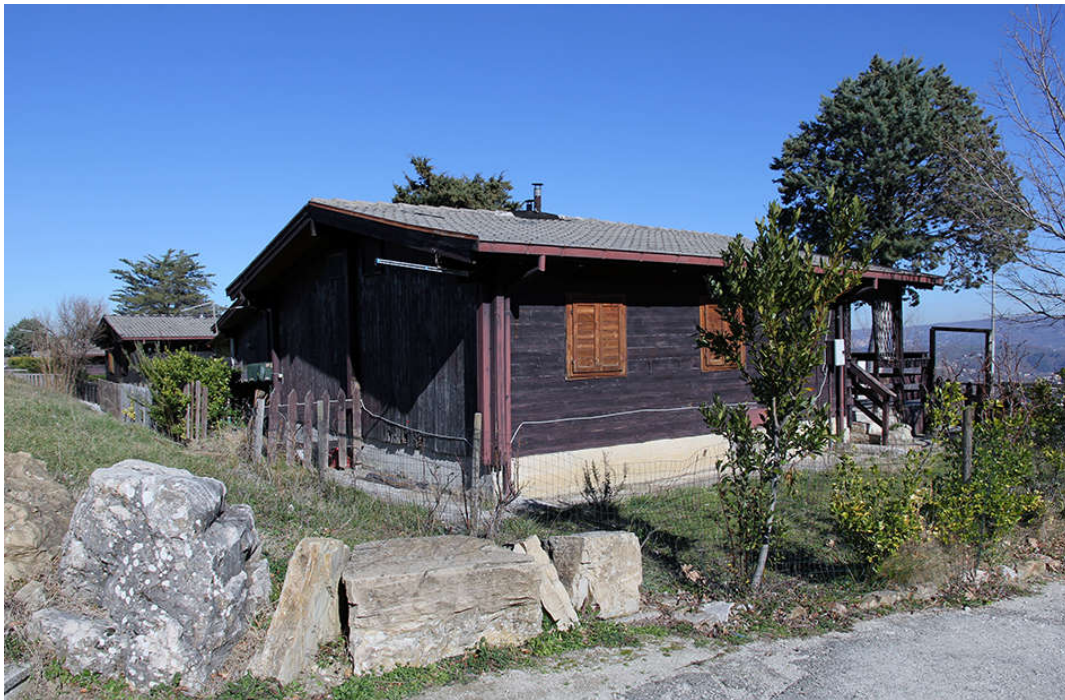
Figure 58. San Mango sul Calore: “Villaggio S. Stefano”. Temporary village, consisting of wooden chalets, built immediately after the 1980 earthquake (photos by [35,36]).
