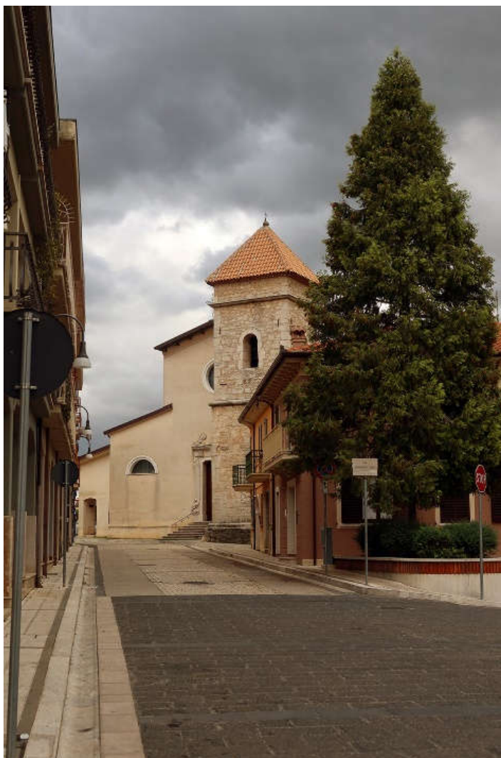
Figure 28. Lioni: restored Church and bell tower of S. Maria Assunta (photos by [35,36]).
