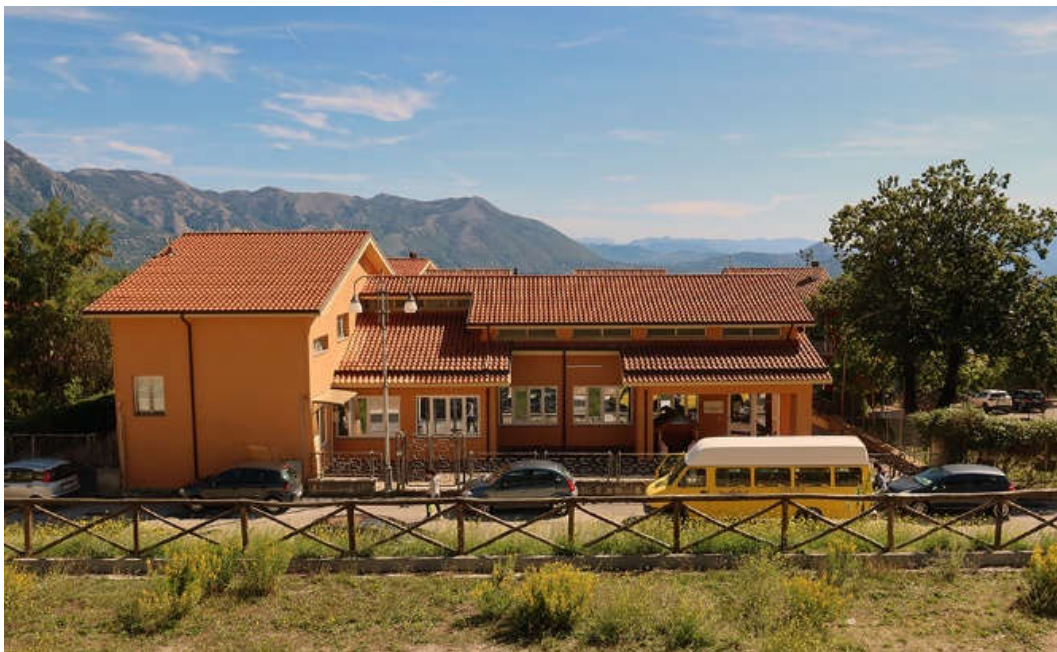
Figure 99. Senerchia: new school complex (photos by [35,36]).
