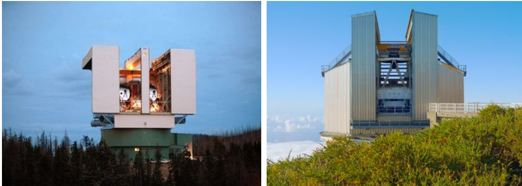
Figure 3.4: Left : LBT, located at Mount Graham, Arizona (USA). It has a binocular design with two identical 8.4 m telescopes. Image taken from https://www.oas.inaf.it . Right : TNG is a 3.58 m telescope located in the island of San Miguel de La Palma (Spain). Image taken from http://tmtlapalma.org/
